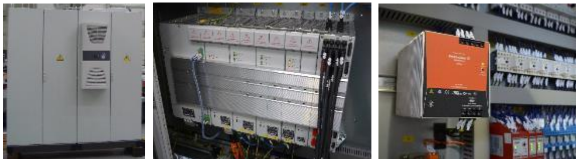
An Example of an Electric cabinet: an Overall View with the Air Conditioning (on the Left), Drives (in the Middle) and Electric Wiring (on the Right)
